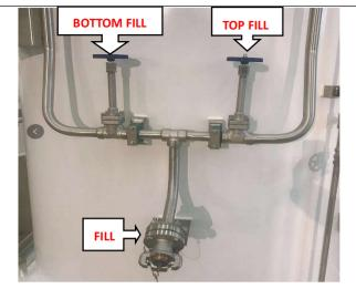
Before first filling, The tank should be cooled with cryogenic First fill, The BOTTOM and TOP FILL valves should be use at the same time. At other times, Only TOP FILL valve should be used when filling.
