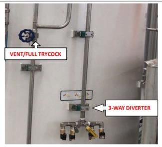
VENT/FULL TRYCOCK valve is used for tank overpressure or Full level discharge
