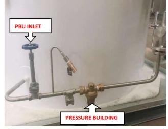
Using, The valve Normally open; If not use, The valve normally close;
