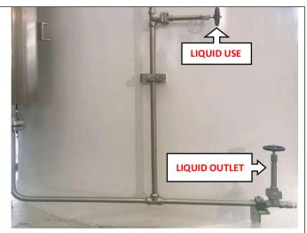
Using, The LIQUID USE VALVE Normally open; Not use, The valve Normally close.
